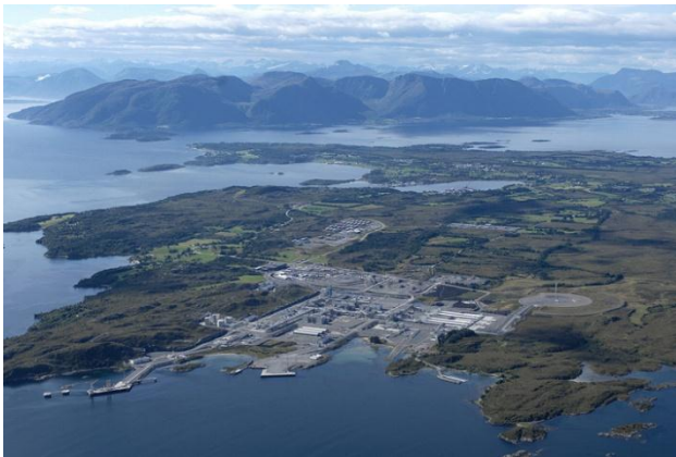
Ormen Lange land plant at Nyhamna
